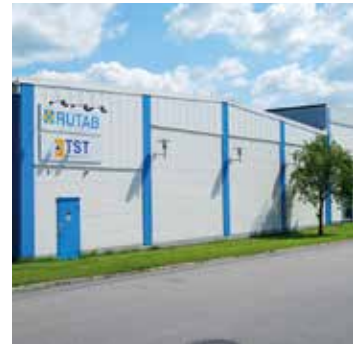
Warehouse - and production facility in Nässjö, Sweden
