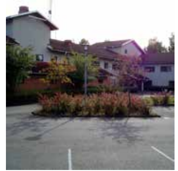
Offices in Nässjö Sweden
